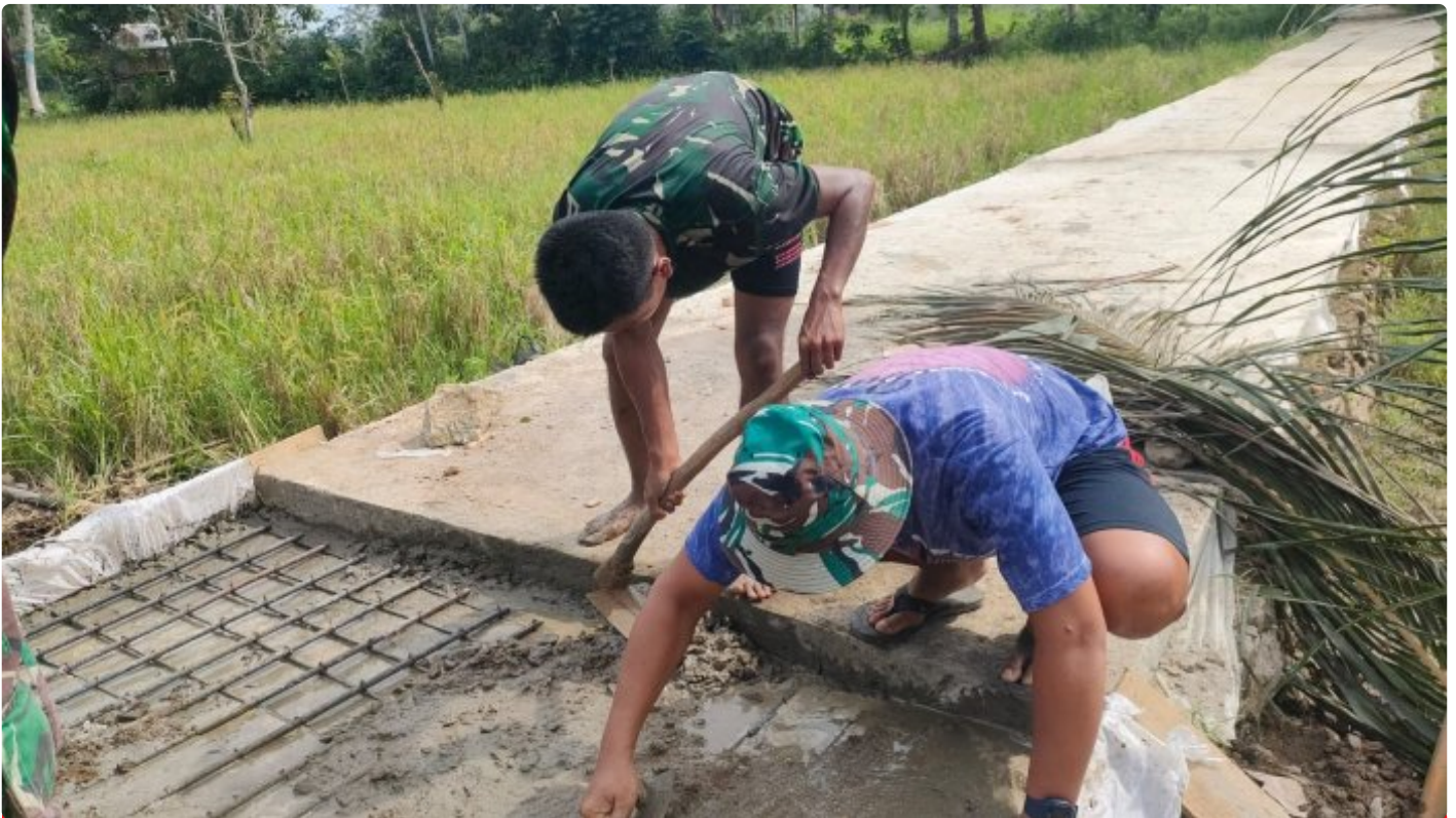
Slop Beton 1 Sasaran TMMD 116 Kodim 1002/HST Capai 60 Persen
